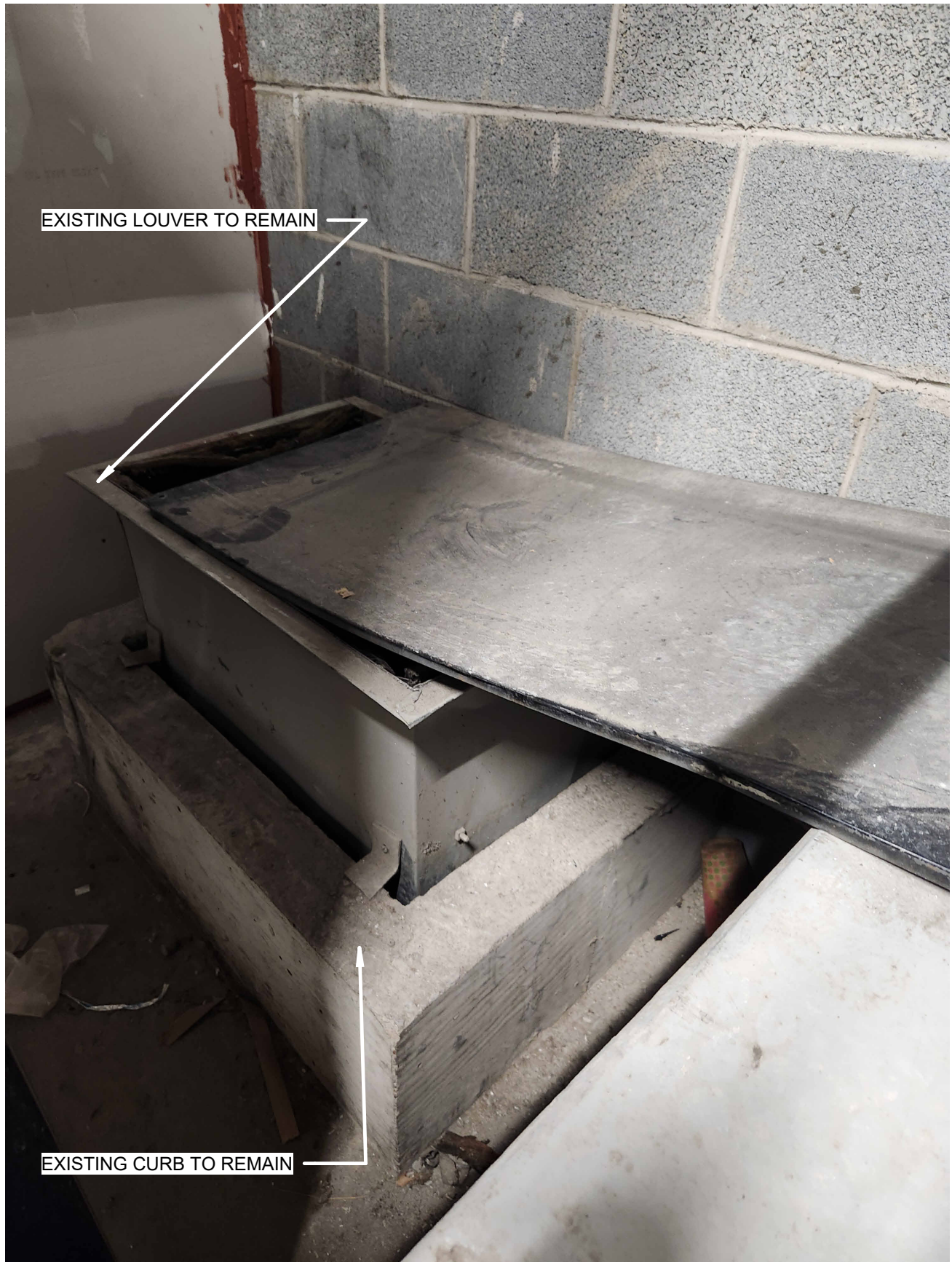
VIEW OF EXISTING FLOOR PENETRATION IN MECHANICAL ROOM
