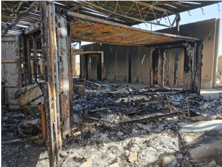
Ruined living quarters at Al Asad (Qiblawi)
